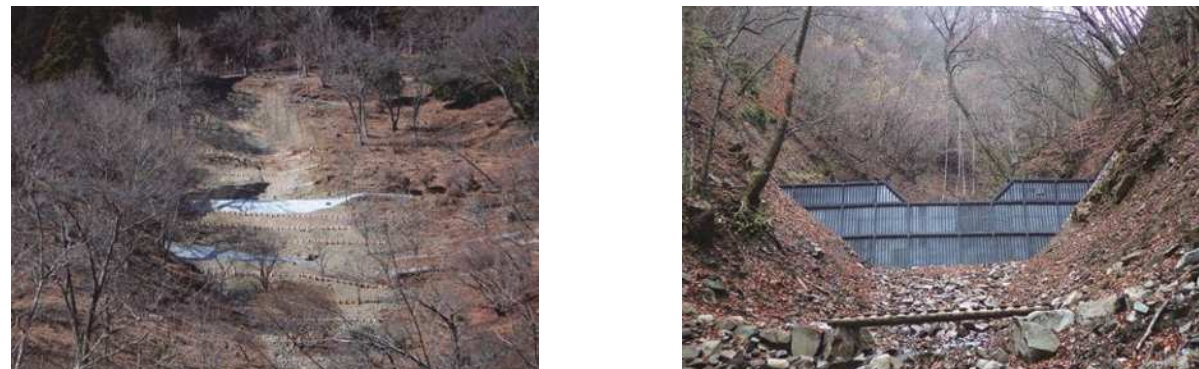
Restoration of landslide areas using the earth retaining wall
