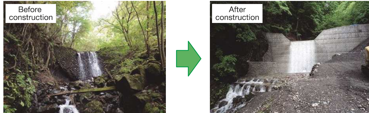
Restoration of erosion control facilities through repairs to damaged sections of check dams
