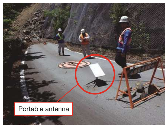
Establishing a communication infrastructure by installing portable antennas
