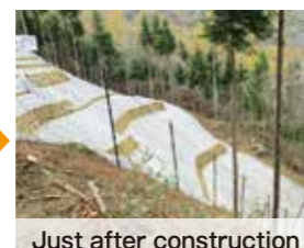
Just after construction
