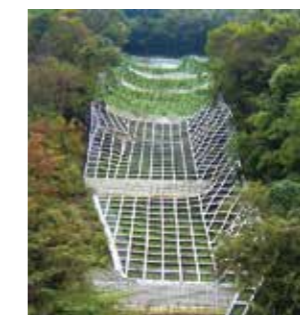
Just after construction
