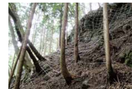
Prevention of rockfall by erosion prevention work
